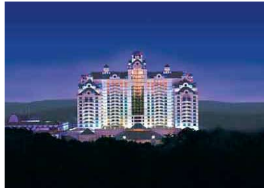
FOXWOODS CASINO PARKING FACILITY Ledyard, Connecticut (Mashantucket Pequot Tribal Nation )
